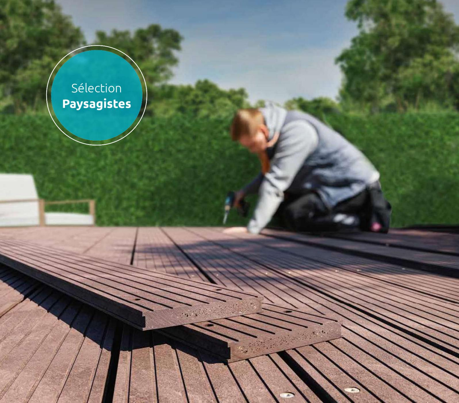
A person in a grey hoodie and dark pants is kneeling on a wooden deck, using a power drill to install a hanit decking board. The deck is made of dark brown, textured wooden planks. In the background, there are green trees and a clear blue sky.
